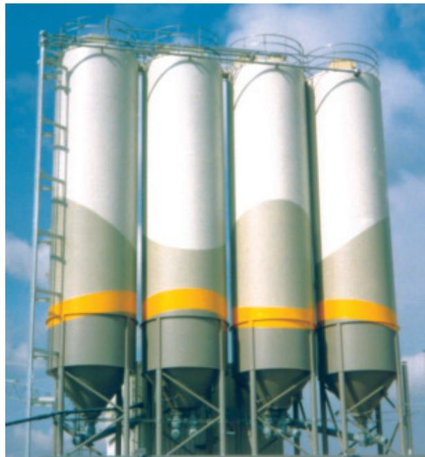
supported by special discharge aids, such as the Stanelle LUALO air injection fluidisation system or the ASK discharge vibrating cone.
